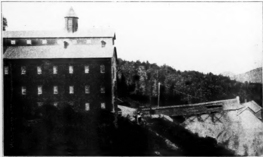
View Showing Mill and Housing for Carrying Waste Materials to Dump
